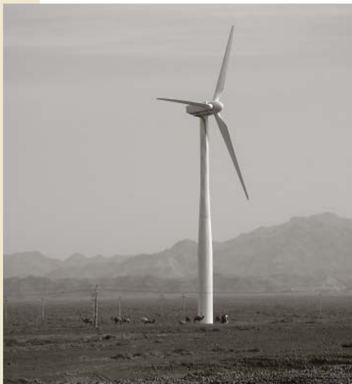
Wind power in western China is a growing energy source.
